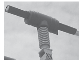
2 Pieces: MVLC-38 on busbar with BCIC
